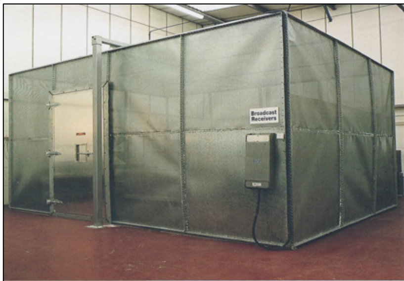
Figure 77 Example of a shielded room made from expanded metal
